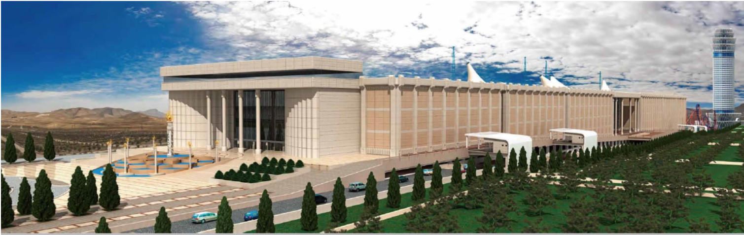
Persian Gulf Commercial Complex (Shiraz, Iran) Total Cooling Capacity: 14,000 USRT (For shopping center only)
