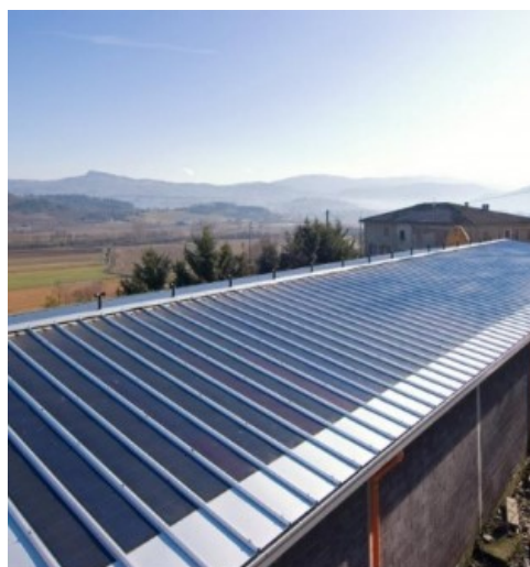
49 kWp Poppi (AR)
